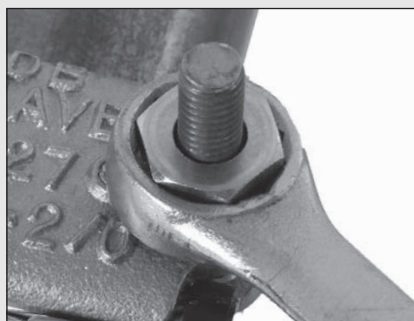
2. Tighten to shear-off hex
